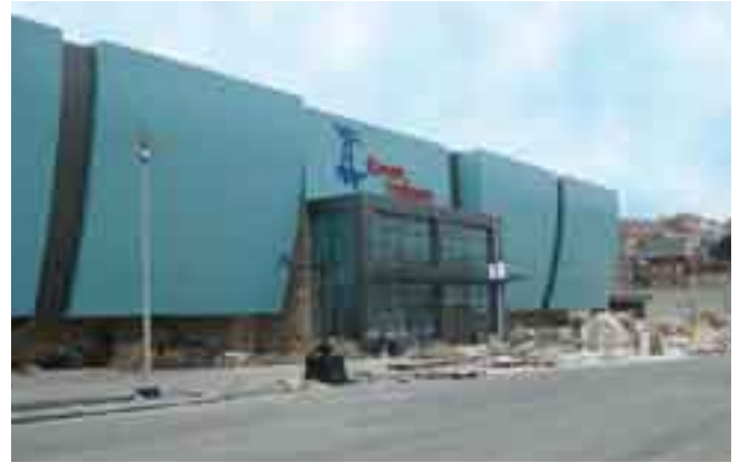
Shopping Centre in Trabzon
